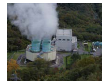
Geothermal Power Plant
